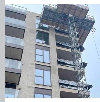
Dansk Boligbyg has just handed over this building, where Combitherms winter mats have been used to protect the railings on the balconies while work was still being done on the upper floors. Photo: Dansk Boligbyg.
